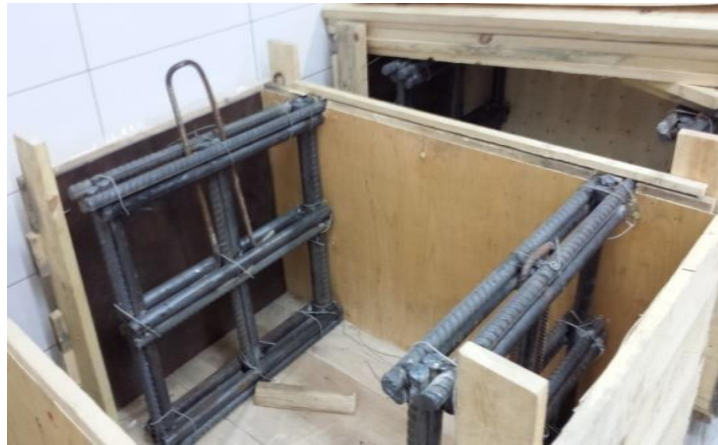
Fig.15. Steel reinforcement for the laboratory RC specimen
