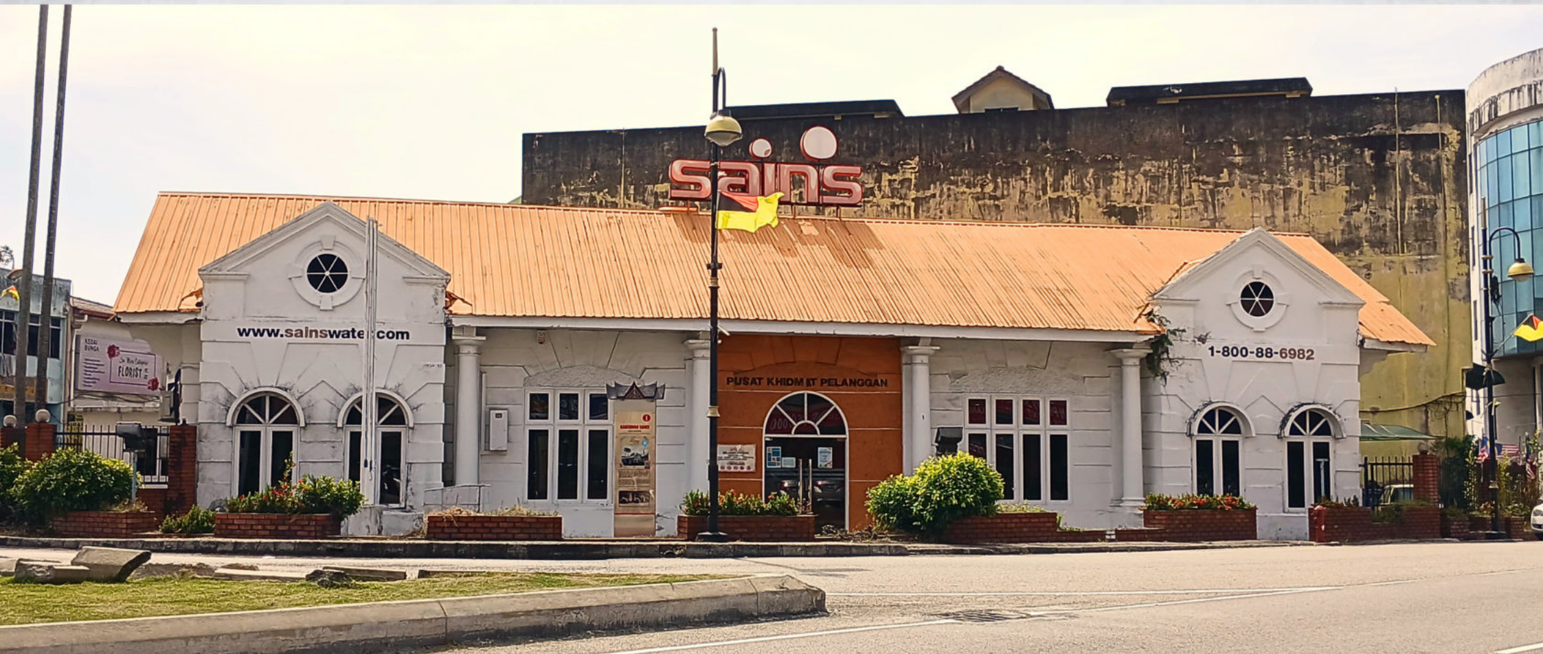
Figure 1.5.1 View of SAINS building
