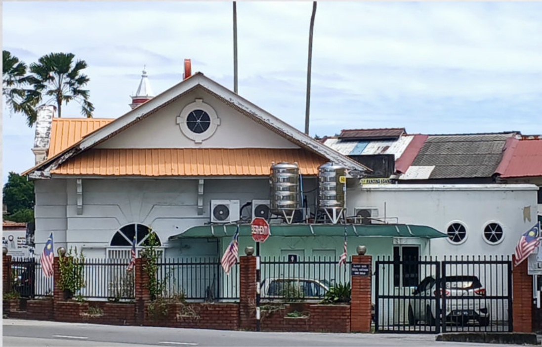
Figure 2.3.2 Rear facade of SAINS Seremban building
