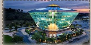
Malaysia Energy Commission Headquarters (ST Diamond Building)
