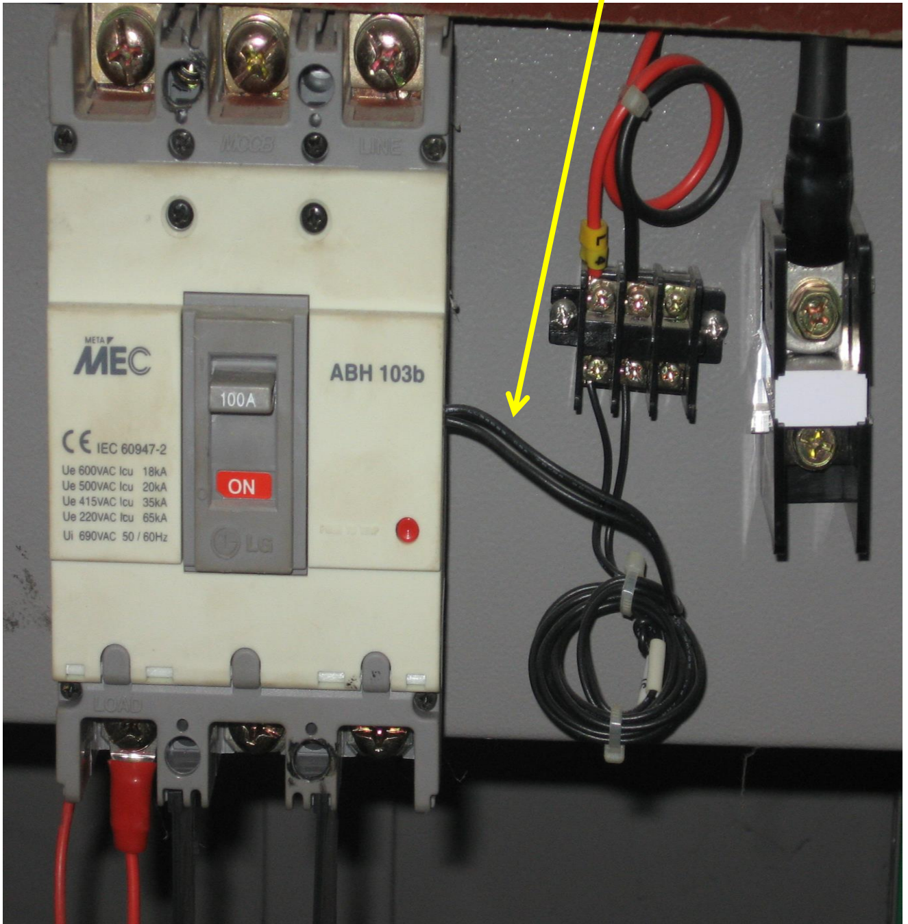
Figure 14: shunt trip coil
