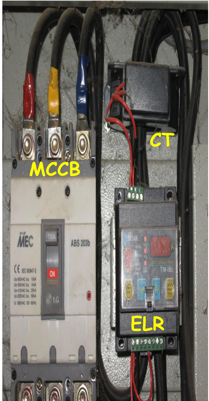
Figure 12: position MCCB, RCCB, CT, ELR in Circuit Breaker
