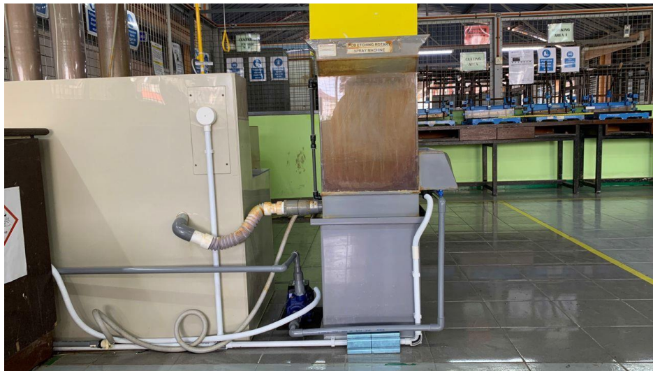
Figure 4: The installation of the motor pump and PVC pipe at the etching machine
