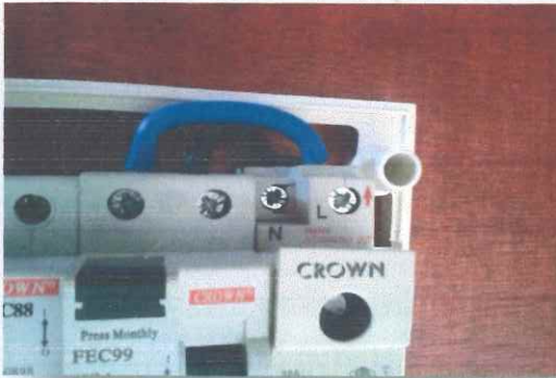
Figure 3.9 : fitting the db board
