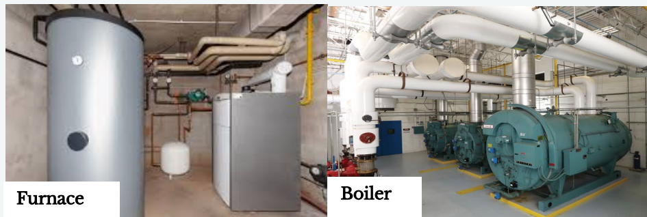
Figure 2.10 Furnace and boiler
