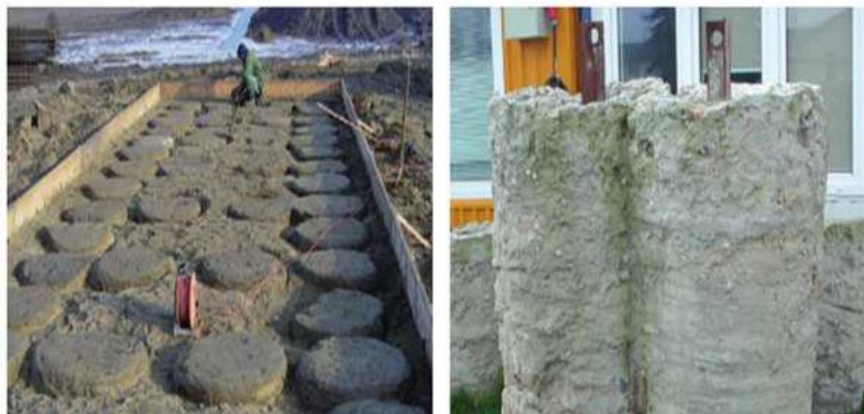
Figure 3.0: Single and extruded overlapping deep mixed soil column (Massarsch and Topolnicki,2005).
