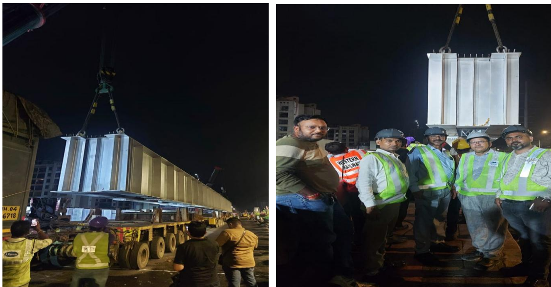
Fig.No.6 Erection(lifting) of Steel Girder
