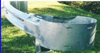
GUARDRAIL TERMINAL (TYPE 2) BULL NOSE
