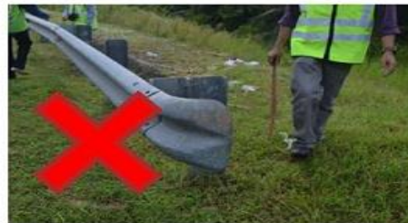
GUARDRAIL TERMINAL (TYPE 1) FISH TAIL
