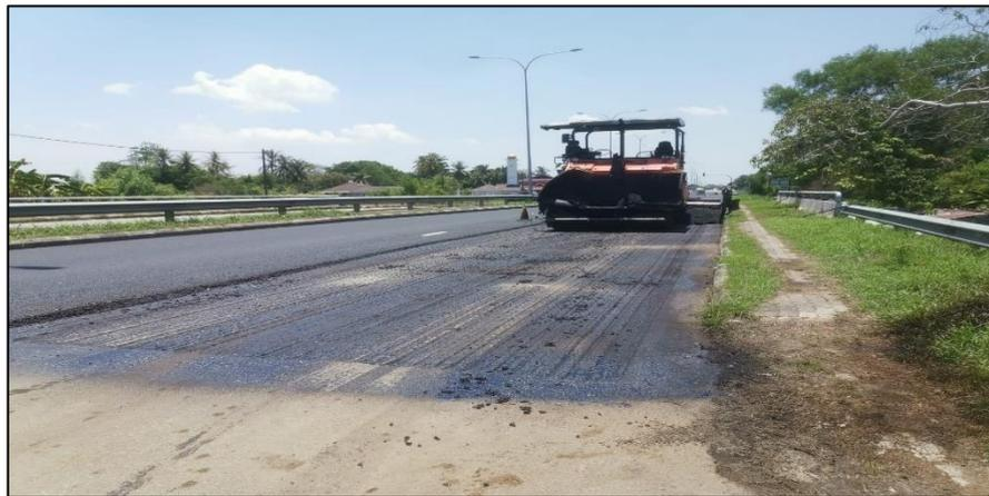
Figure 1.1 : Shortages of material at the end of section
