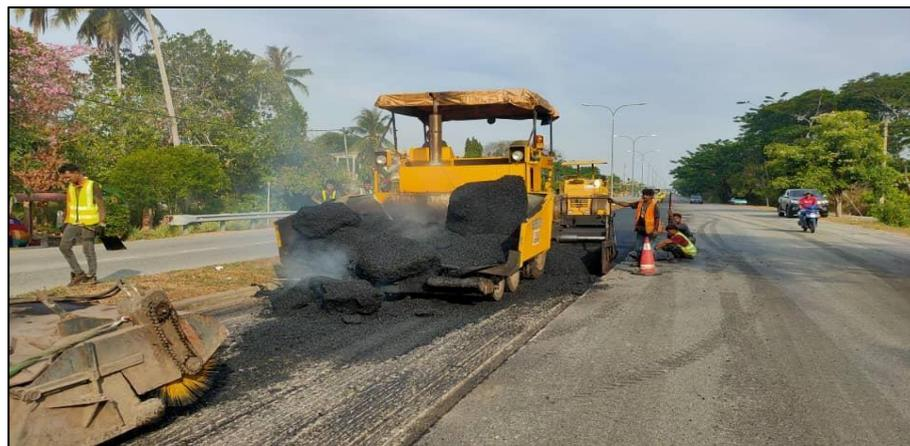
Figure 1.2 : Large lump of premix due to delay on site
