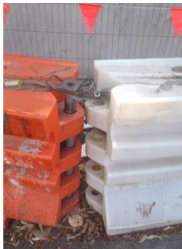
Figure 2.10: Example of pin connection.
