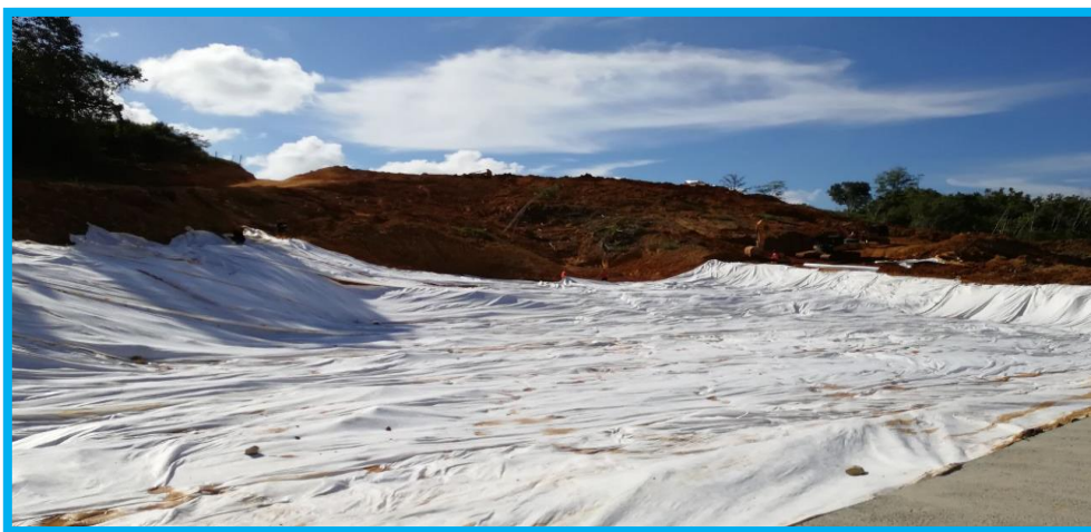
Figure 2.1: Placement of geotextile in soil treatment
