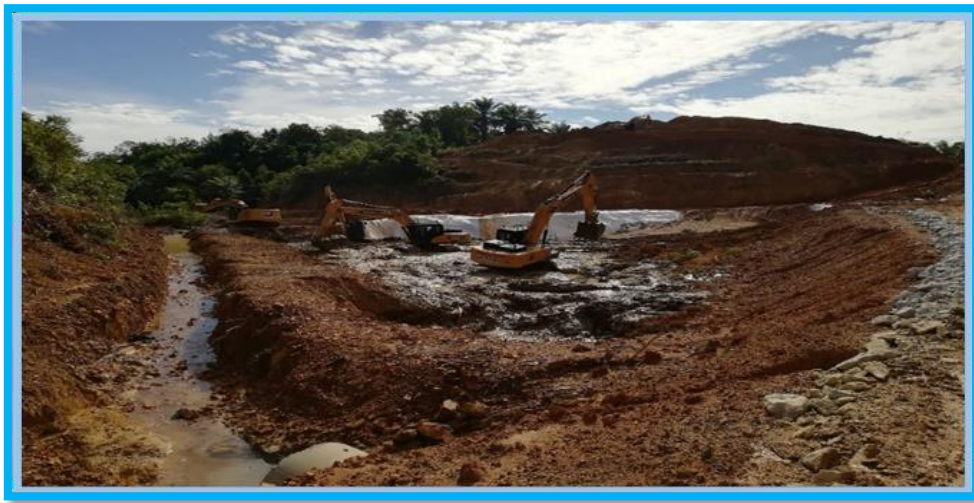
Figure 1.2: Remove and Replace Method in Setiu, Terengganu
