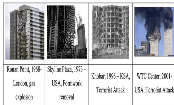
Fig. 13. Some historical buildings subjected to progressive collapse.
