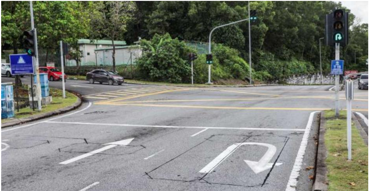
Diagram 2.2.1: Common Traffic Light Sensor
