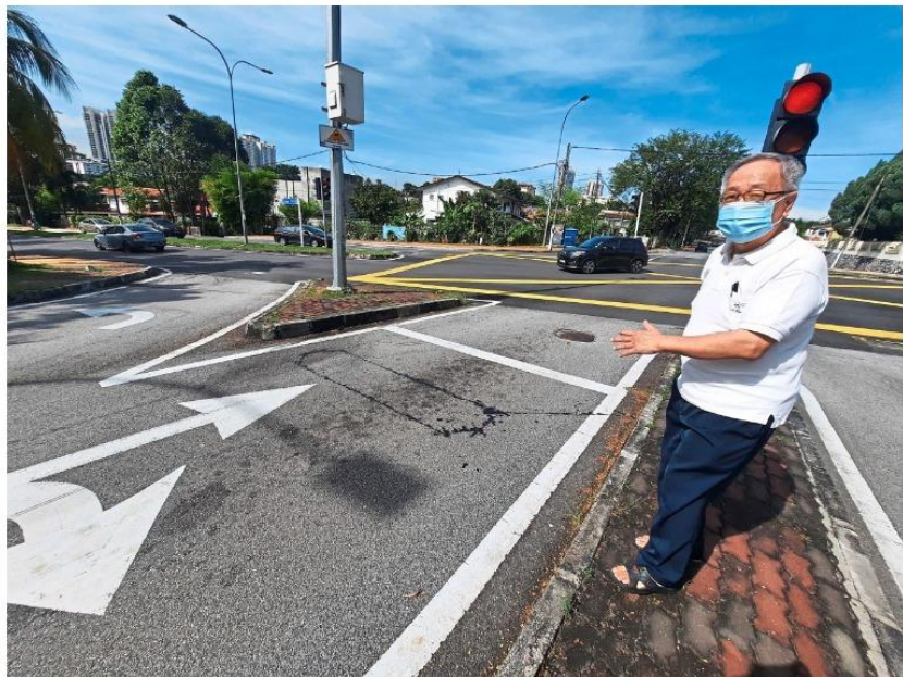
Wong showing the white line on the cross junction at Jalan 16/6. Motorists need to stop on the line to activate the sensor.
