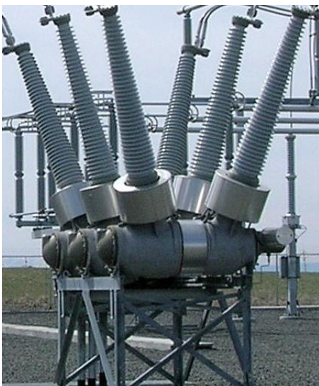
Figure 2.15 : SF 6 Circuit Breaker
