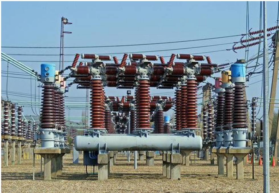
Figure 2.19 : Air-Blast Circuit Breaker.
