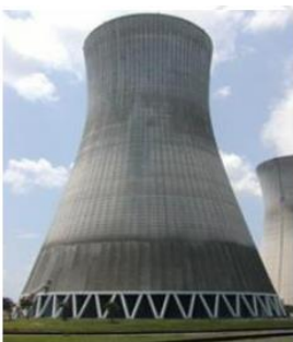
Natural Draft Cooling Towers
