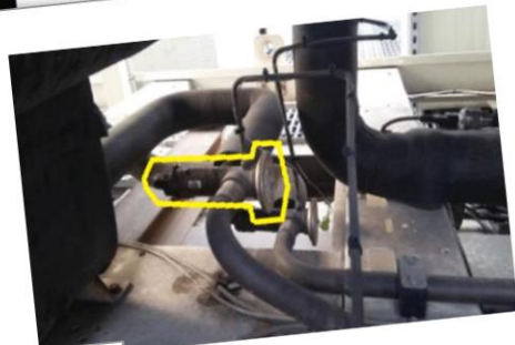
Thermal expansion valve
