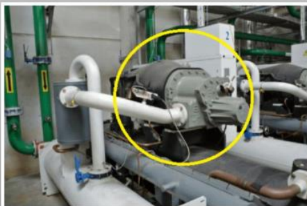
Screw type compressor
