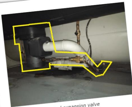
Pilot operated thermal expansion valve
