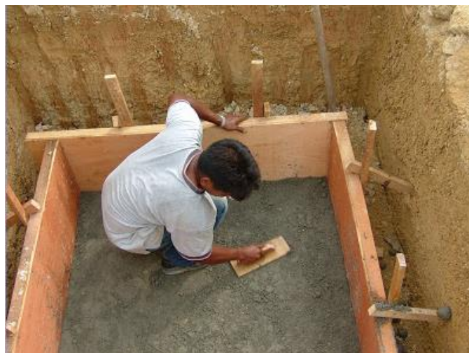
Rajah 30: Kerja-kerja meratakan lean concrete
