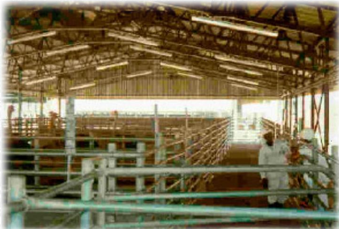
Fig 15: Smooth tubular rails for pens partition
