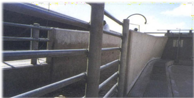
Figure 9 : Installation of solid side on ra ces
