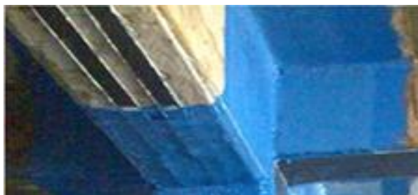
Fig -8: After strengthening
