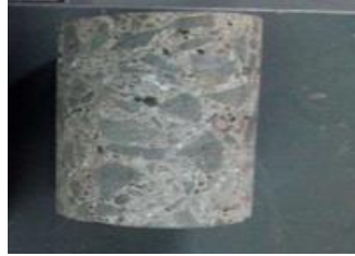
Figure 5: Core test sample of Beam 01
