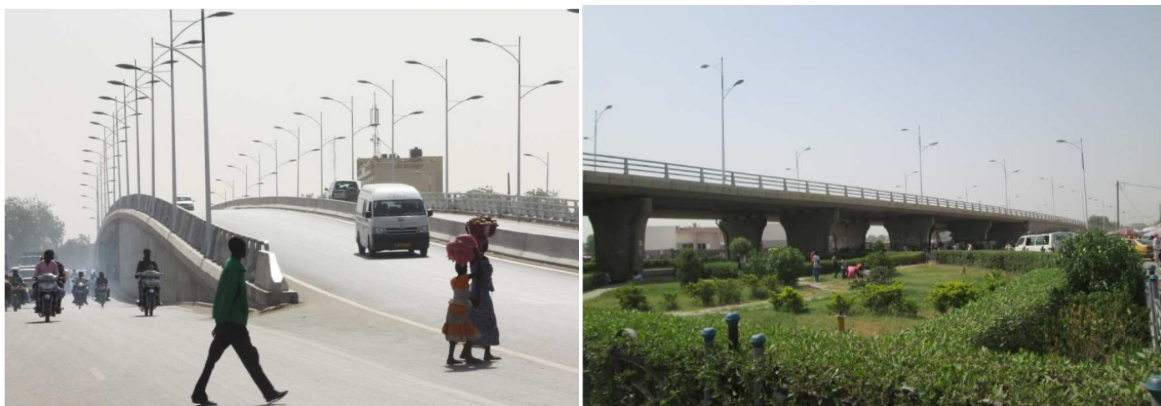
Image 1: The Dembé and Diguel viaducts
