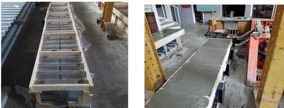
Figure 3. Casting of concrete
