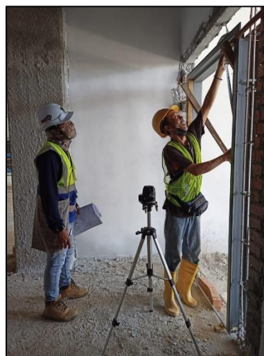
Figure 2.1: Installation Door Frame
