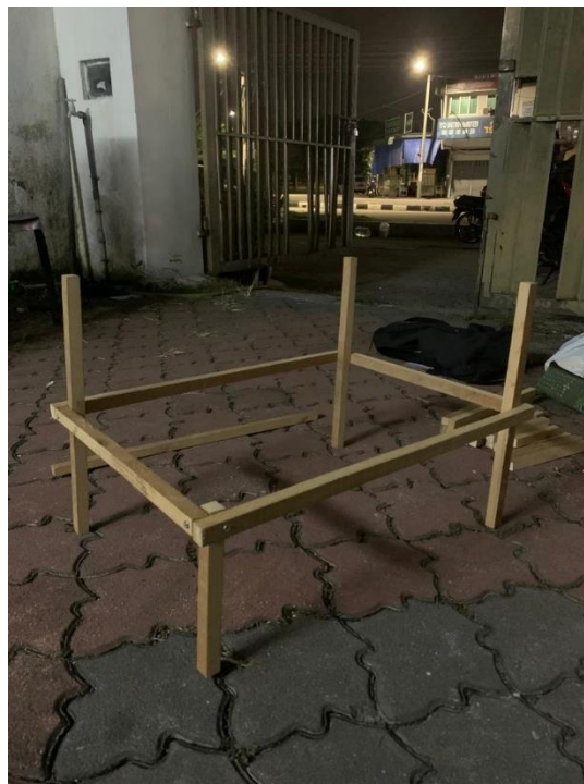
Figure 3.30: Assembling the frame
