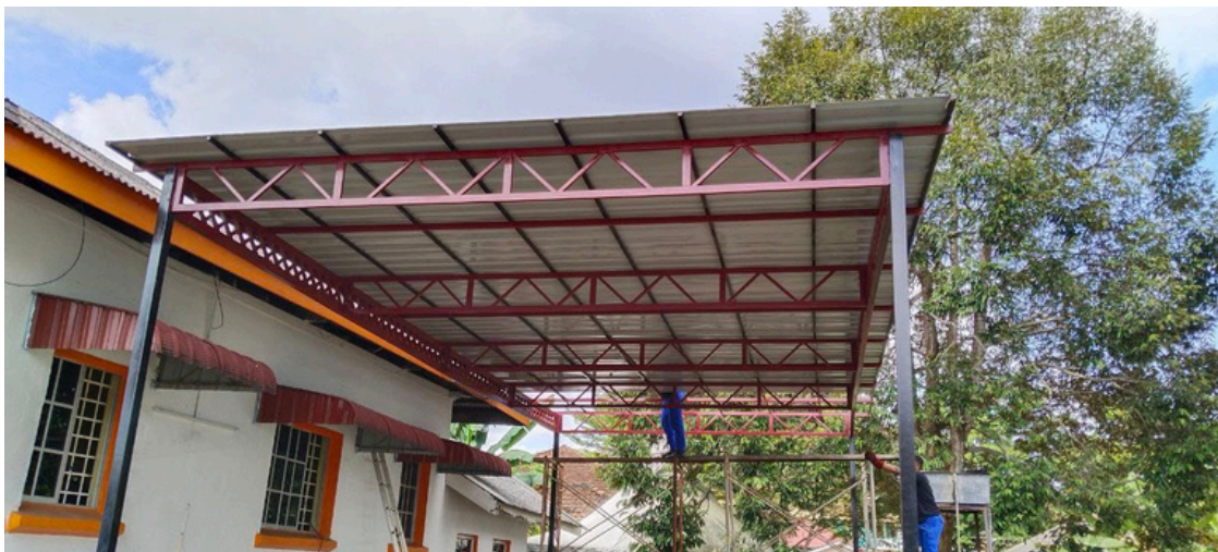
Rajah 20 Kursus Shielded Metal ARC Welding SMAW For Fillet Weld 4F.
