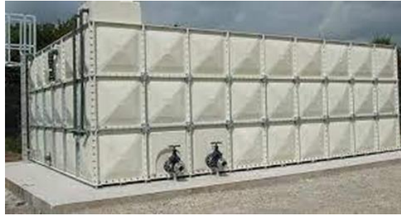
Figure 2.1: Fiberglass Reinforced Plastic Water Tank
