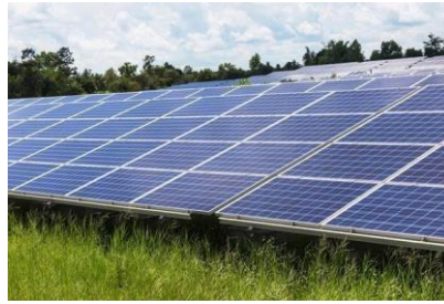
Figure 2.10: Polycrystalline solar panel
