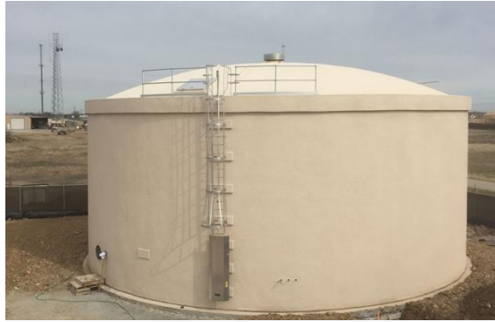
Figure 2.5: Concrete Water Tank
